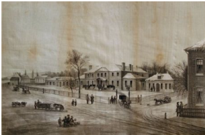
Figure 1. View of Province Hall and Public offices, Fredericton, destroyed by fire. Completed in 1802, Province Hall. (Permission for use: New Brunswick Provincial Archives MC300-MS18 from the York-Sunbury Historical Society Collection.) This picture is of a lithograph by George Smith c 1850. From left to right, 1790 house and business of Peter Fraser, the Anglican Church, and the 1816 stone government structures on either side of province hall.
